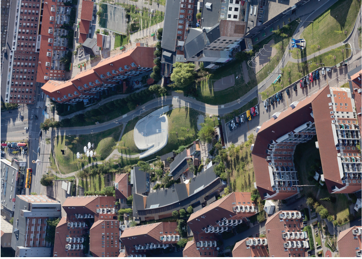
Superkilen, 2012. Green Park. Photo: Iwan Baan.
