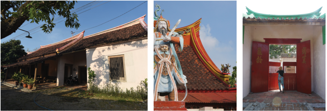
From left to right: the swallow-tail roof made of terracotta still survives at the residence of Captain Lim Ki Siong. Photo: Feri Latief. The roof of Cu An Kiong Temple. Photo: Astri Apriyani. The gate shaped like a swiftlet roof, and the courtyard floor made of terracotta. Photo: Agni Malagina.
