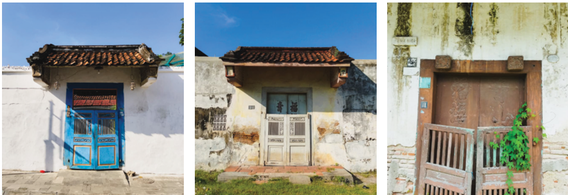
The house gates and fence walls are made of terracotta; the gate and door leaf design is unique because it differs from that of gates in Quanzhou; the use of Chinese characters on the gateway is unusual in Quanzhou, yet used in Lasem. Photo: Agni Malagina.
